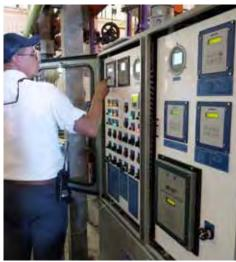
Altronic Controls panels that CIC installed automatically control the blower valves, as well as fuel switching for the engines. The main Altronic components are a DE-3000 Safety Shutdown System with CPU-95 Ignition, DET-1600 Detonation and Misfire Sensor, EZRail, EPC-150 with dual-fuel stepper valves, and VSM Vibration Sensing Monitoring System. Woodward 2301D and DCL catalyst were also installed. The next planned
